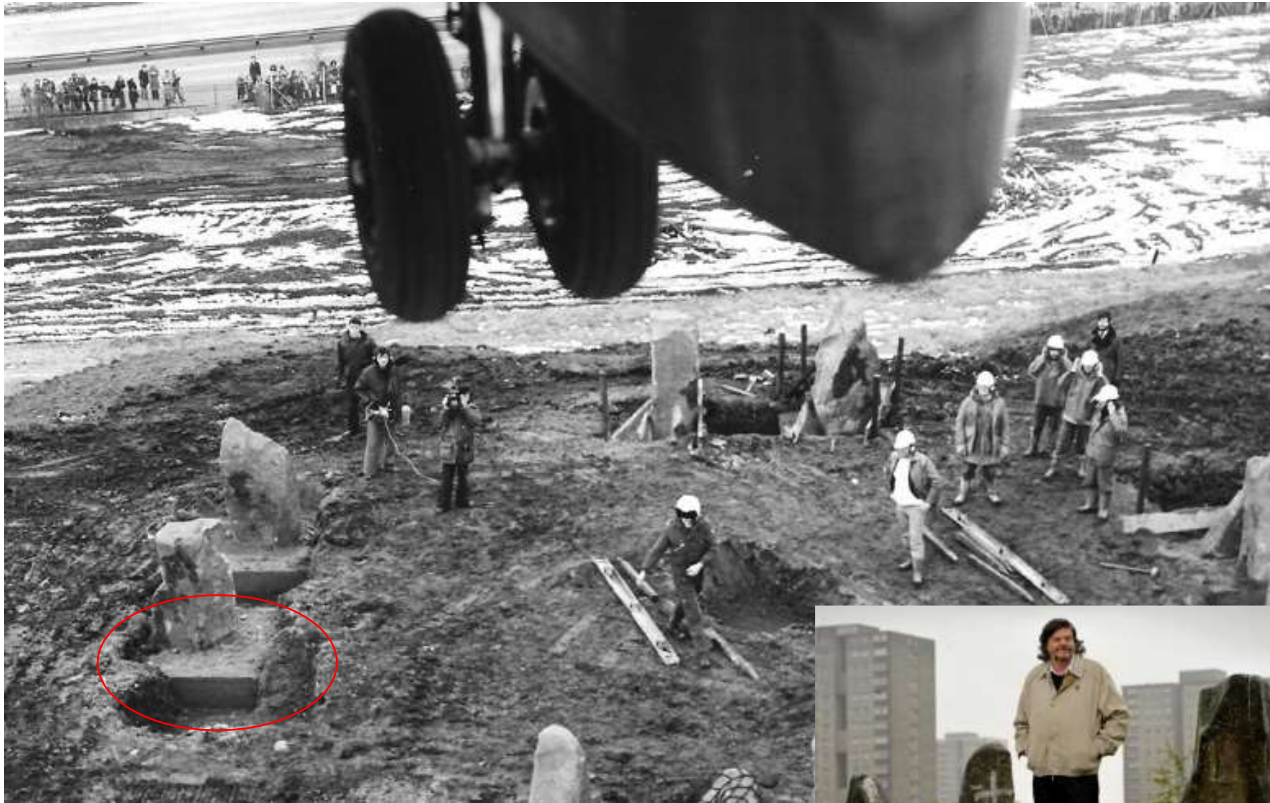
Construction of the circle in 1979, and Dunan Lunan (right)
