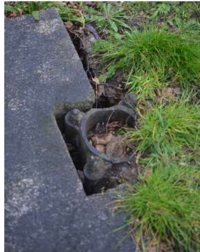
Figure 2.2 Scraps of a mega event: the socketed base of one of the Crystal Palace's cast-iron columns at Sydenham today. Source: Photograph by the author.
